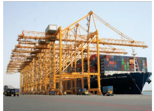
Ship to shore cranes.
