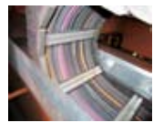
Guide channel installation
