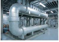
This heat exchange system cools our injection molding equipment with heat from an electrical generator.
