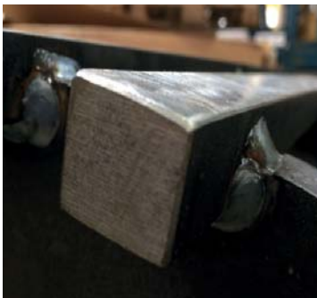
Close up of finished steel bar
