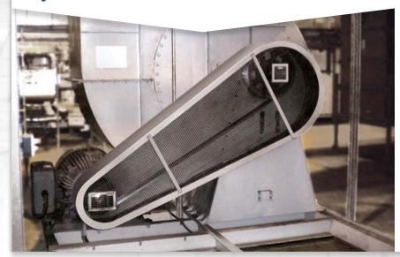
The ventilation systems in the "THORP" reprocessing plant at Sellafield in England are liable to be exposed to high temperatures. Conventional drive belts used in these systems suffered frequent failures as a result. Unplanned maintenance in such a sensitive environment is highly undesirable, so in 2010, after advice from Optibelt's engineers, the operator began equipping his plant with optibelt RED POWER maintenance-free wedge belts.
