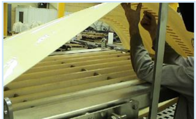
Belt repaired on site.
