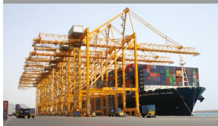
Cranes and hoisting
