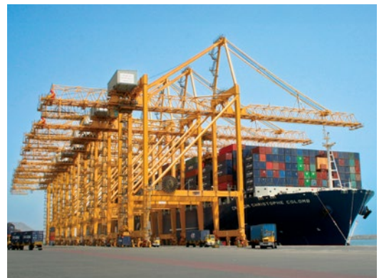
Ship to shore cranes.
