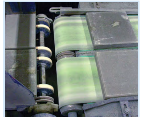
FK - 3 Brick pre - oven conveying
