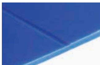
Butt welding with paddle welding tool
